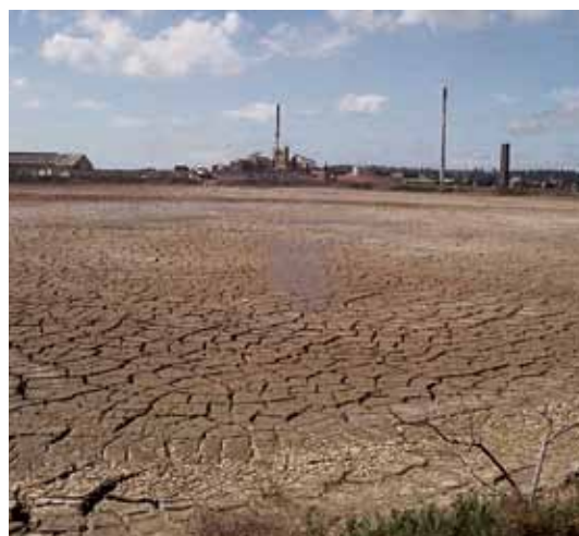
Effluent precipitation and settling dams, after closure.
